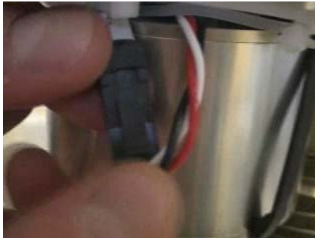
Figure 19 -- Black, red, and white motor phase-leads as connected.
