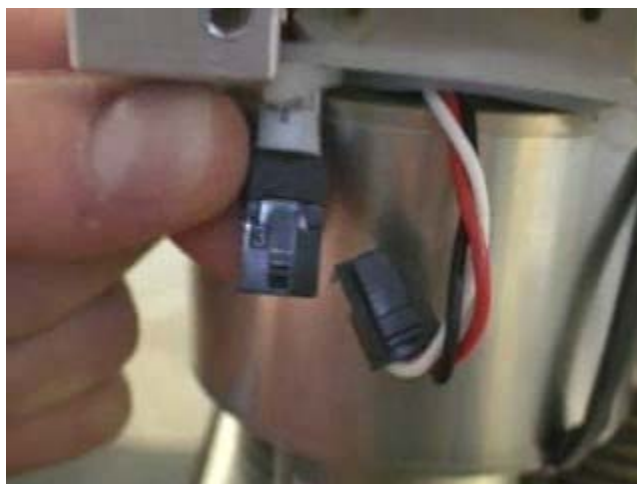
Figure 20 -- Phase leads disconnected.
