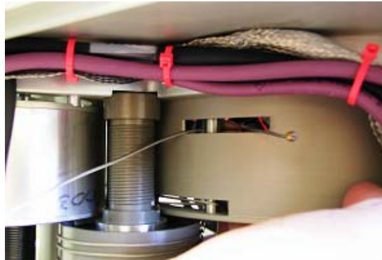
Figure 31 – Looping Cable around the Inboard Stage-2-Pulley Termination Post
